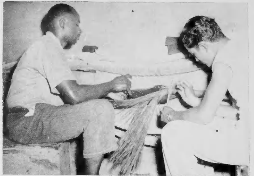
As part of the expansion of the new telephone facilities, D. Mitchell and G. Arends splice cable in the refinery.
